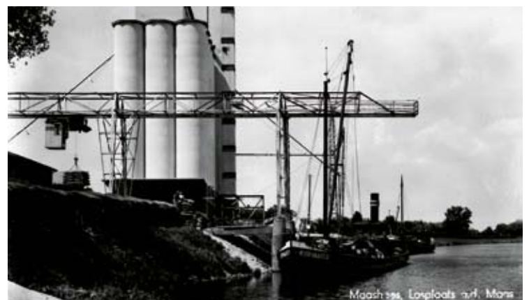
The first silo in 1939. It was destroyed in WW II (1944) and rebuilt in 1948/49.
